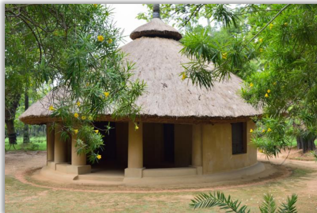
Figure 9: Small mud and coal tar house called Chaitya in Shantiniketan: Sustainable living.
