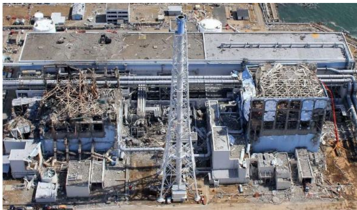
Figure 17. The damaged reactor units of Fukushima Daiichi Nuclear Power Plant. (Source: The New York Times)
