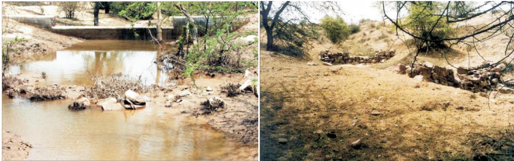
Figure 8. Check dam made from (A) masonry work and (B) loose stones (Source: Ref. 8).
